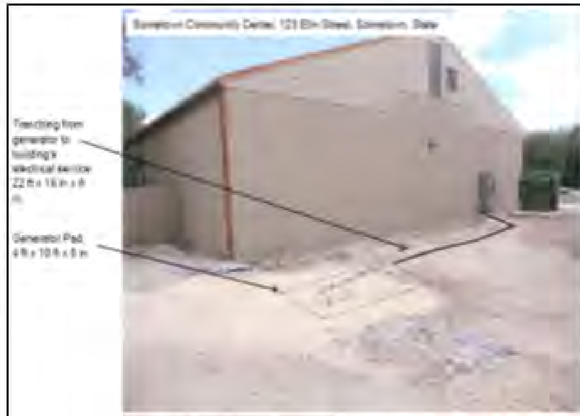
Figure 4. Ground-level photograph showing proposed ground disturbance area.
